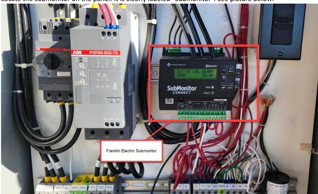
4. Once the submonitor has been located on the lower right portion of the submonitor frame, the serial number is located See pictures below.
